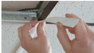
Applying GridMax™ Over T-bar Suspension Grid System
