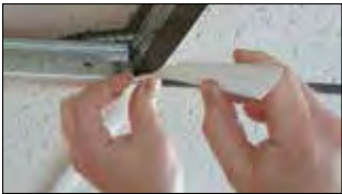
Applying Gridmax over T-bar suspension grid system
