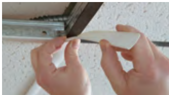
Applying GridMax™ Over T-bar Suspension Grid System
