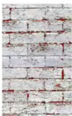
BRICK WALL, PEELING PAINT
