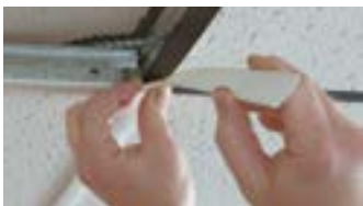
Applying GridMax™ Over T-bar Suspension Grid System
